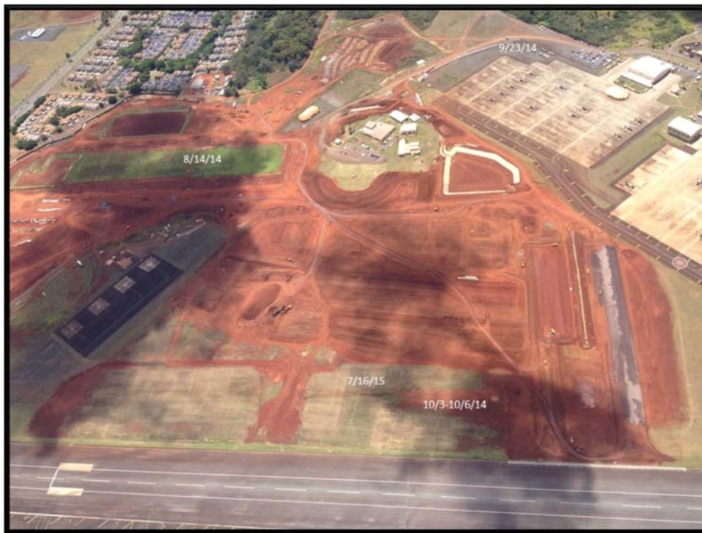
Figure 11: Aerial photo of the WAAF construction site.
